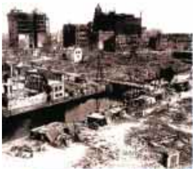
Left: The devastation of Tokyo in 1923 by a fire that broke out after an earthquake measuring 8.3 on the Richter scale.
