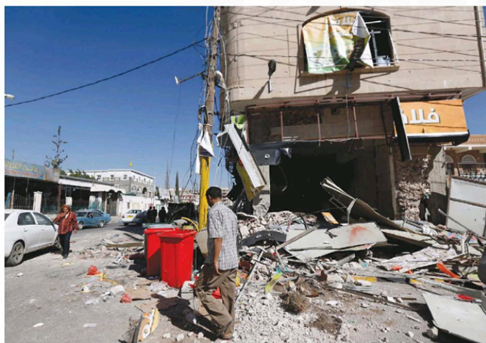
A MAN walks passed a destroyed building in Yemen's Sanaa. (Reuters)
